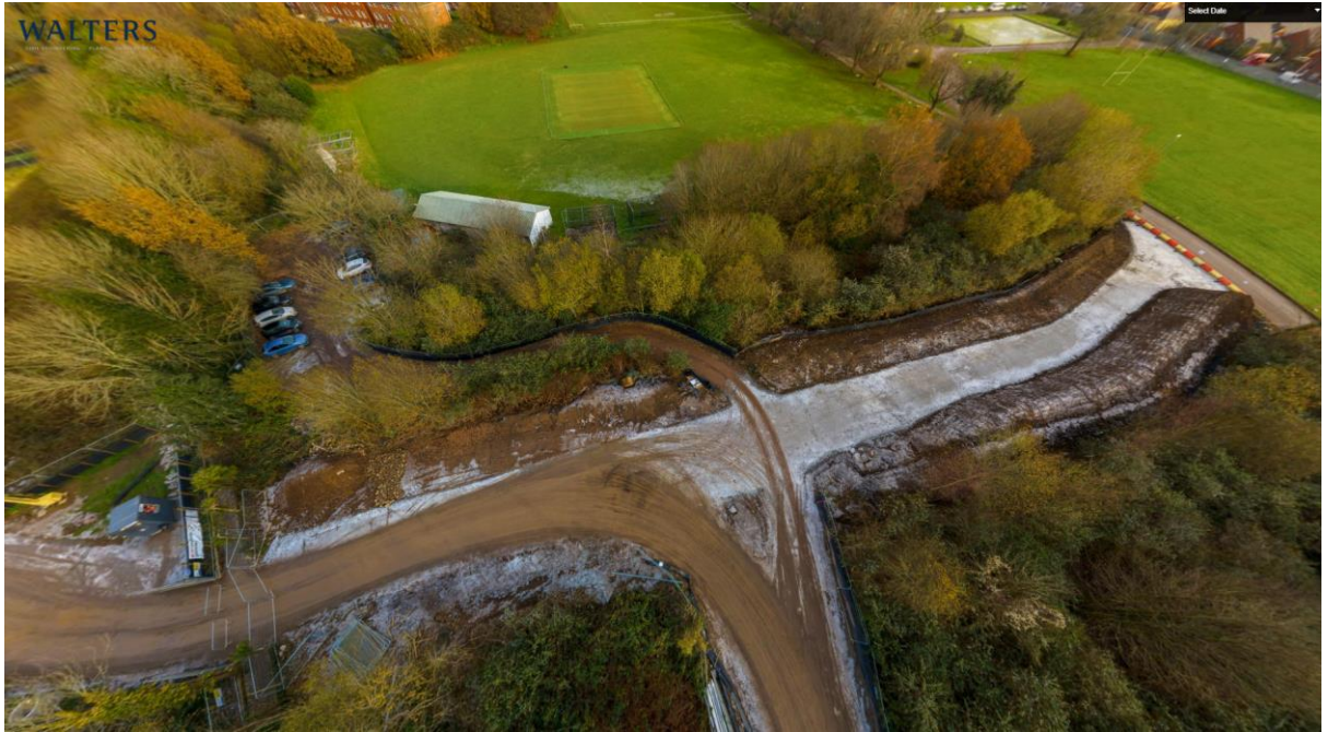
Figure 3: Aerial Photograph of Site Showing Access during Construction (December 2012)
